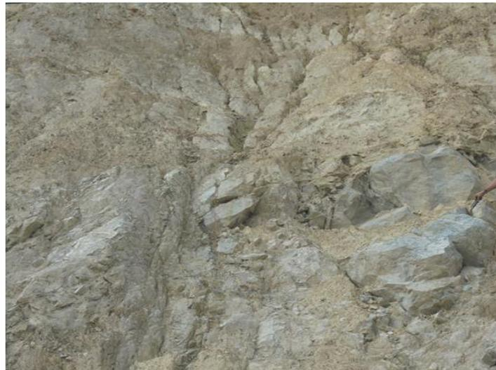
**FOTOGRAFÍA 94. SURCOS SOBRE TALUD DE CORTE ESTACION CL 020 E: 826.167 N: 1.170.144, CARRETERA QUE COMUNICA LAS VEREDAS LA ESTRELLA Y BERMEJAL (SECTOR FINCA LA MANUELA)**
